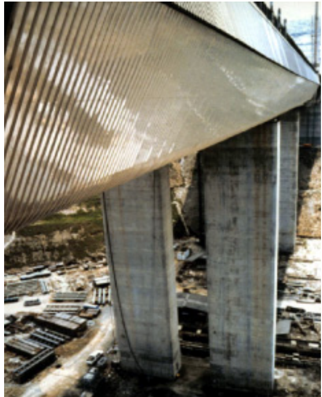
Tsing Ma Bridge, Hong Kong Mott MacDonald 316/2D
