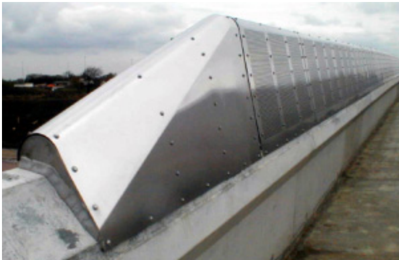
Channel Tunnel Rail Link Kent, England Bridge parapet covers
