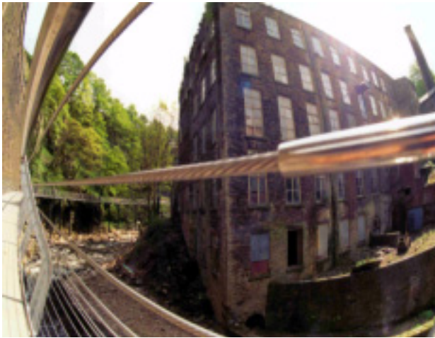
Elevated Walkway Goyt Valley, Derbyshire, England Derbyshire Consulting Engineers 316
