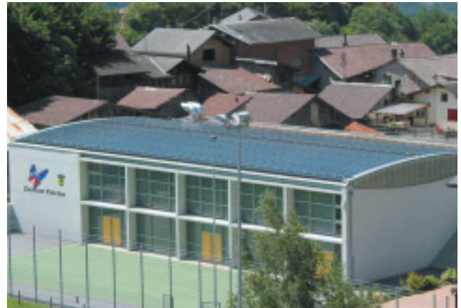
The solar roof of the Varen (Switzerland) sports centre (Photo: Energie Solaire SA)
