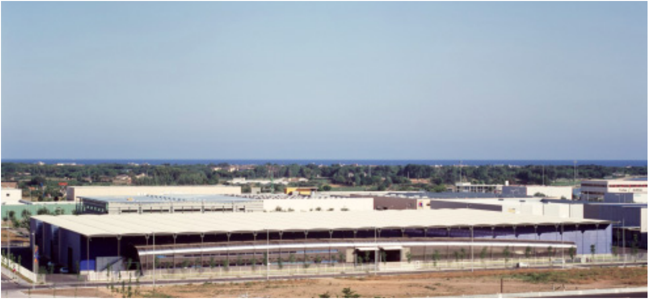
Location of the complex within the Camí Ral industrial estate
