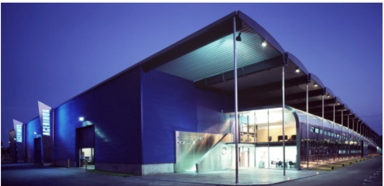
Stainless steel downpipes lend rhythm to the facade
